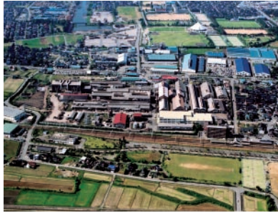
Higashi - Toyama, Steel Plant
